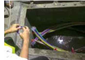
Smaller ducts and handholes
