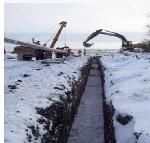
Open Trenching in cold weather Microduct- DB Aluminum
