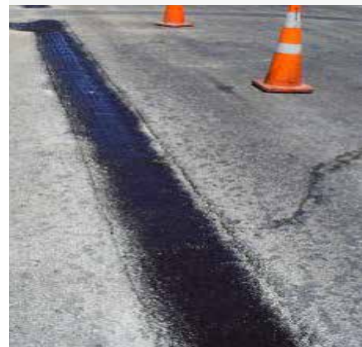
Backfill of Micro trenching Microduct- Link Duct
