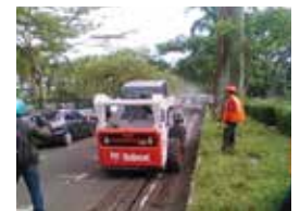
Cut by Micro trencher Indonesia Bandung Municipal project
