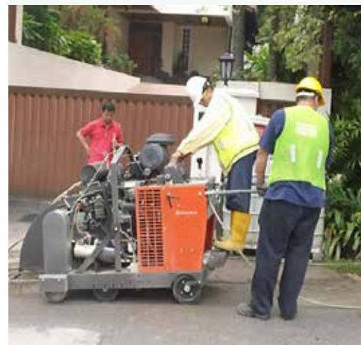
Micro-trenching Microduct – Flat Duct
