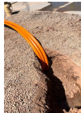
The bundled assemblies enter the bore together, creating 21 independent pathways.
