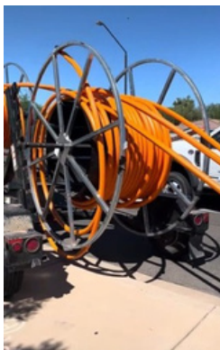
Three 7-way 18/14mm bundled-microduct reels are staged for installation.
