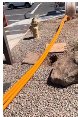
Three bundles approach the bore entry point as one coordinated installation.
