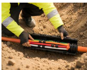
Microduct splice closures are designed to simplify fiber deployment and maintenance while providing long-term reliability. Compared to direct burial splicing, closures keep connections protected, organized, and easily accessible for future use.
